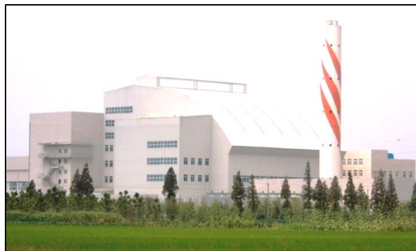
Shanghai, China, waste-to-energy , BOOT, 18 MWe
