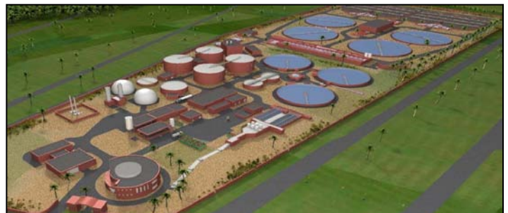
Marrakech (Morocco) – Biotim® wastewater treatment plant with energy production and water re-use
