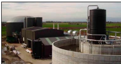
Valmass, Belgium, biomass to energy and wastewater treatment
