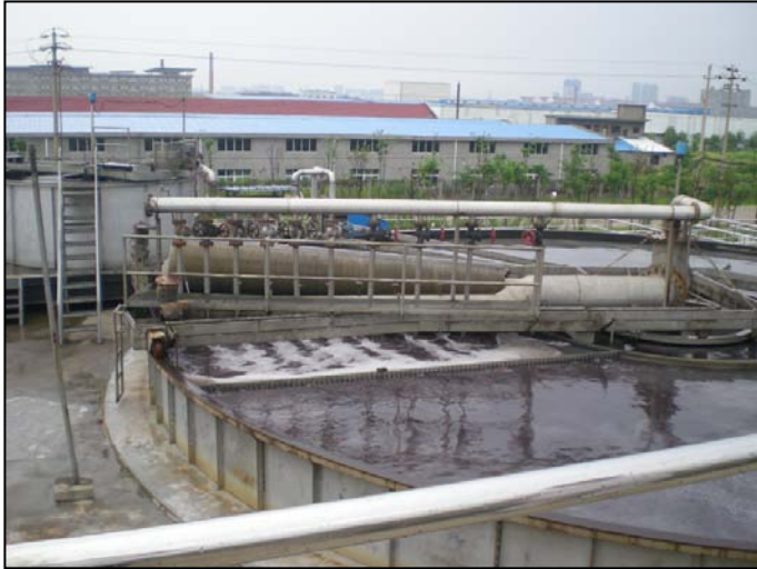
The treatment process at this plant is by way of Sequential Batch Reactor (SBR) and uses RWT's in-house proprietary equipments.
