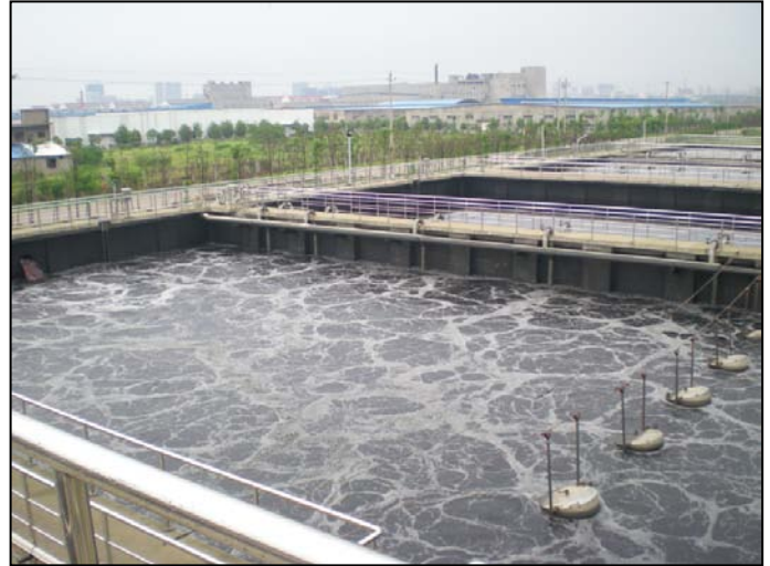
The treatment process at this plant is by way of Sequential Batch Reactor (SBR) and uses RWT's in-house proprietary equipments.
