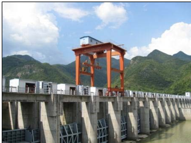
Wuliting Plant, Zhejiang Province Capacity: 42MW
