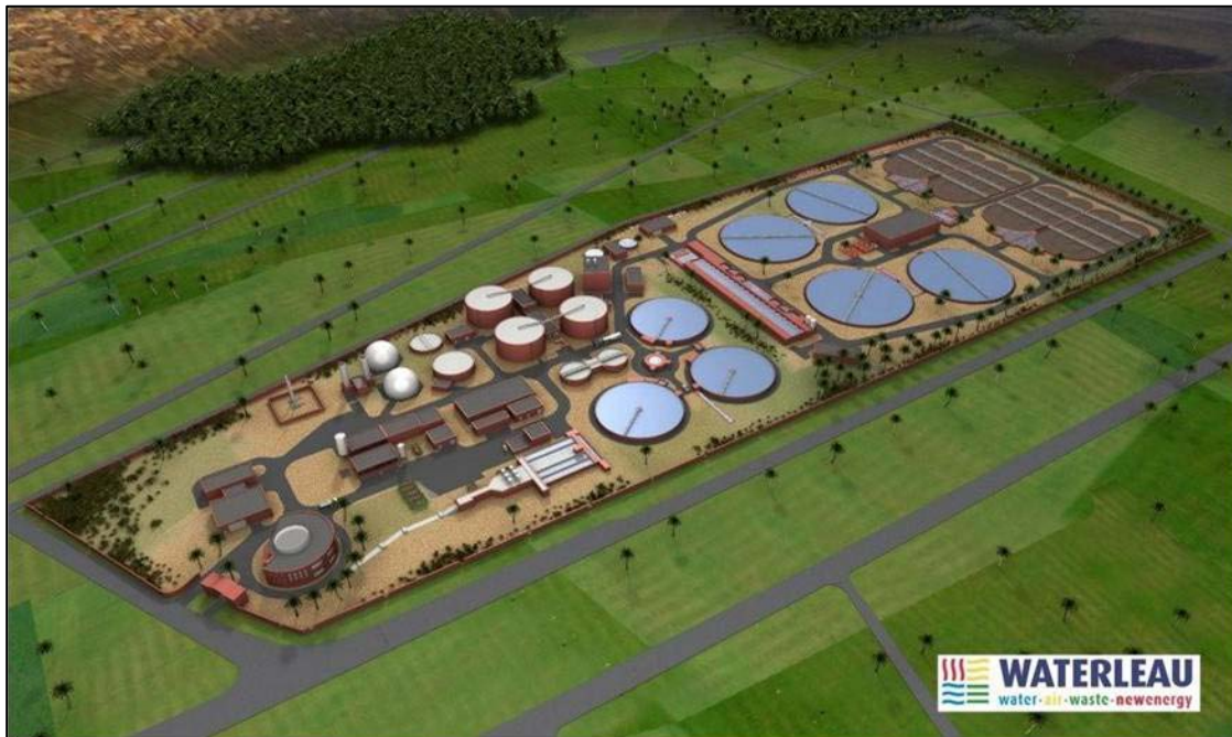
Marrakech (Morocco) – Biotim® WWTP with energy production and water reuse
